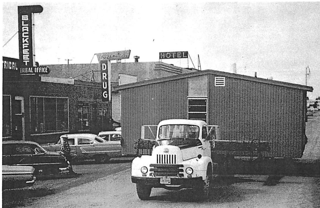
A NEW HOME for a flood refugee family is hauled down Browning's main street. More than 125 homes were destroyed or damaged beyond repair, and are being replaced.
